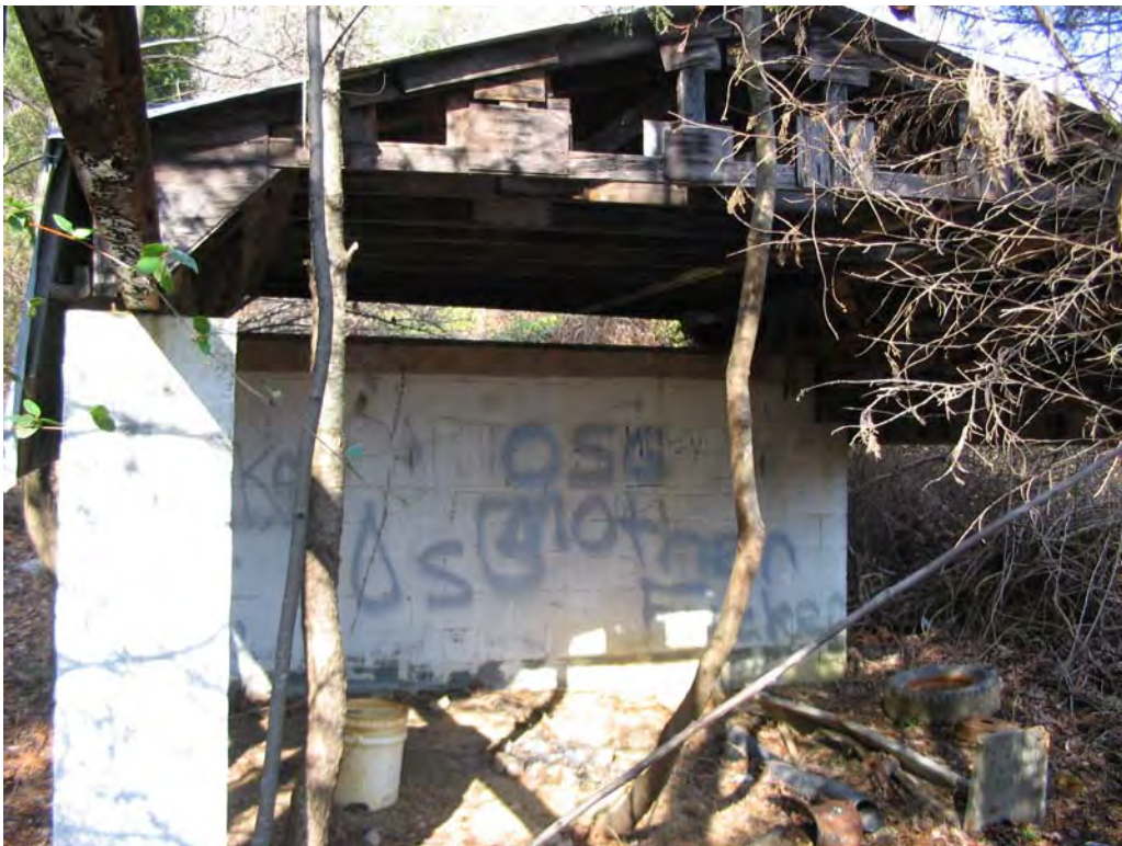
PLATE 10 Building 1, South Elevation, Facing North
